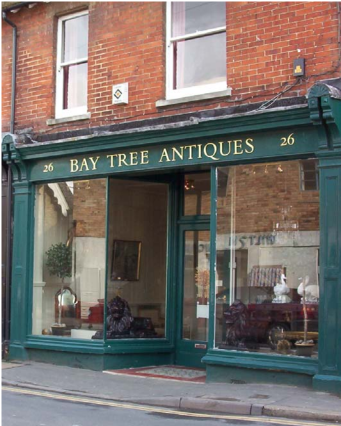
Fig 3: An example of a traditional recessed doorway. Decorative Victorian floor tiles survive in the entrance 'foyer'.
