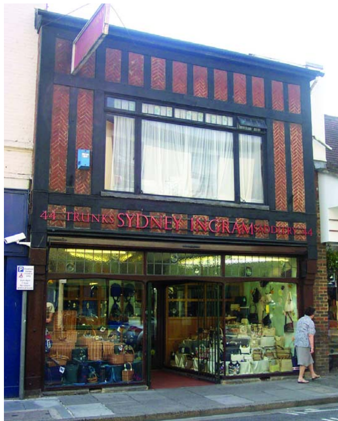
Fig 4: Another example of a recessed doorway. The glass of the shopfront is divided by the Arts and Crafts style leaded lights, which also reflect the style of the building above. There is no fascia so the lettering is applied directly to the building in the fascia position.
